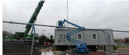
Our temporary buildings have been put in place
